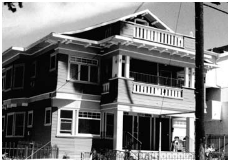
H. J. Moline Flats on Monte Vista St. received a 2004 HPHT award for a façade and restoration.
